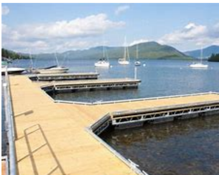
Figure 15: Example of dock facility
