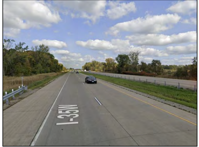
Looking northwest on Interstate 35W (Google street view)
