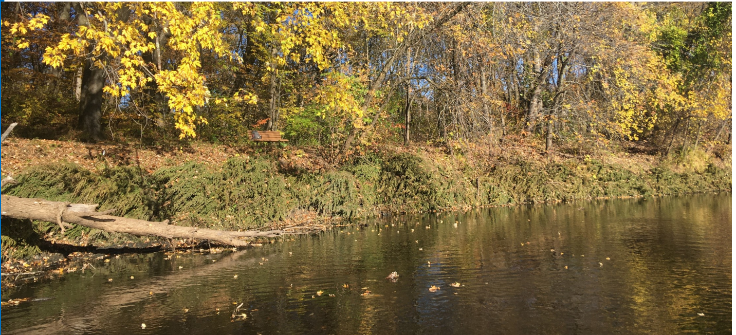
Cedar trees providing soft armoring to a moderately eroding bank in Rum Central Regional Park. This erosion was threatening a trail.
