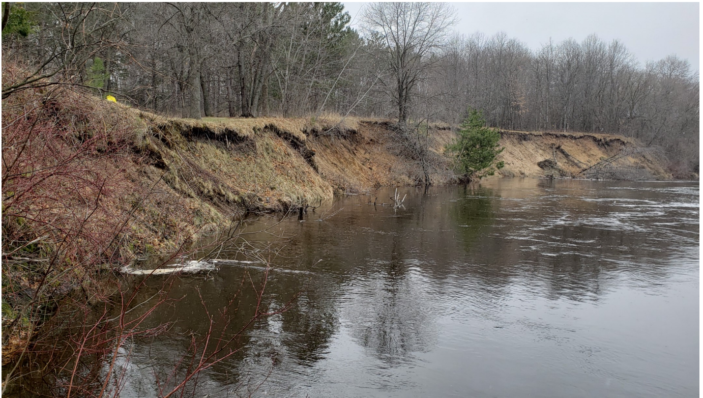
The 400+ foot project we are working towards stabilizing in Oak Grove
